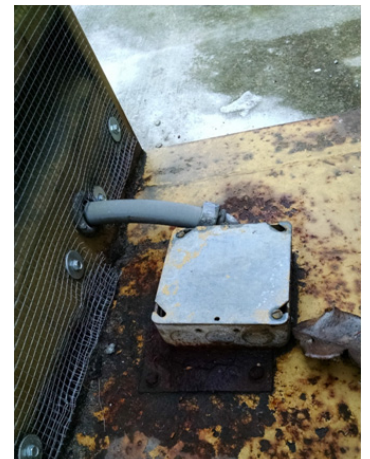
A single-wall tank and the level sender electrical box is exposed to the weather. Water is getting into the tank.
