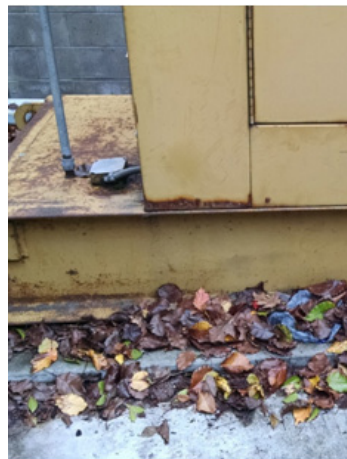
A single-wall tank and the level sender electrical box is exposed to the weather. Water is getting into the tank.
